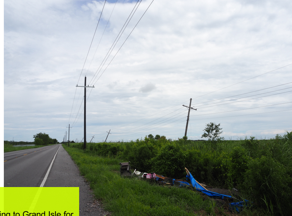
Figure 10: Old Poles and New Poles, 2022
