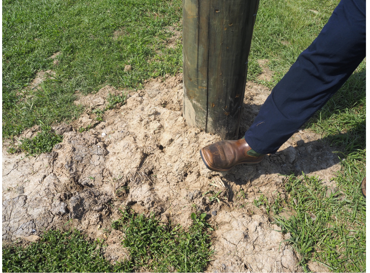
Figure 6: Pole with Dried Clay at Base, 2022
