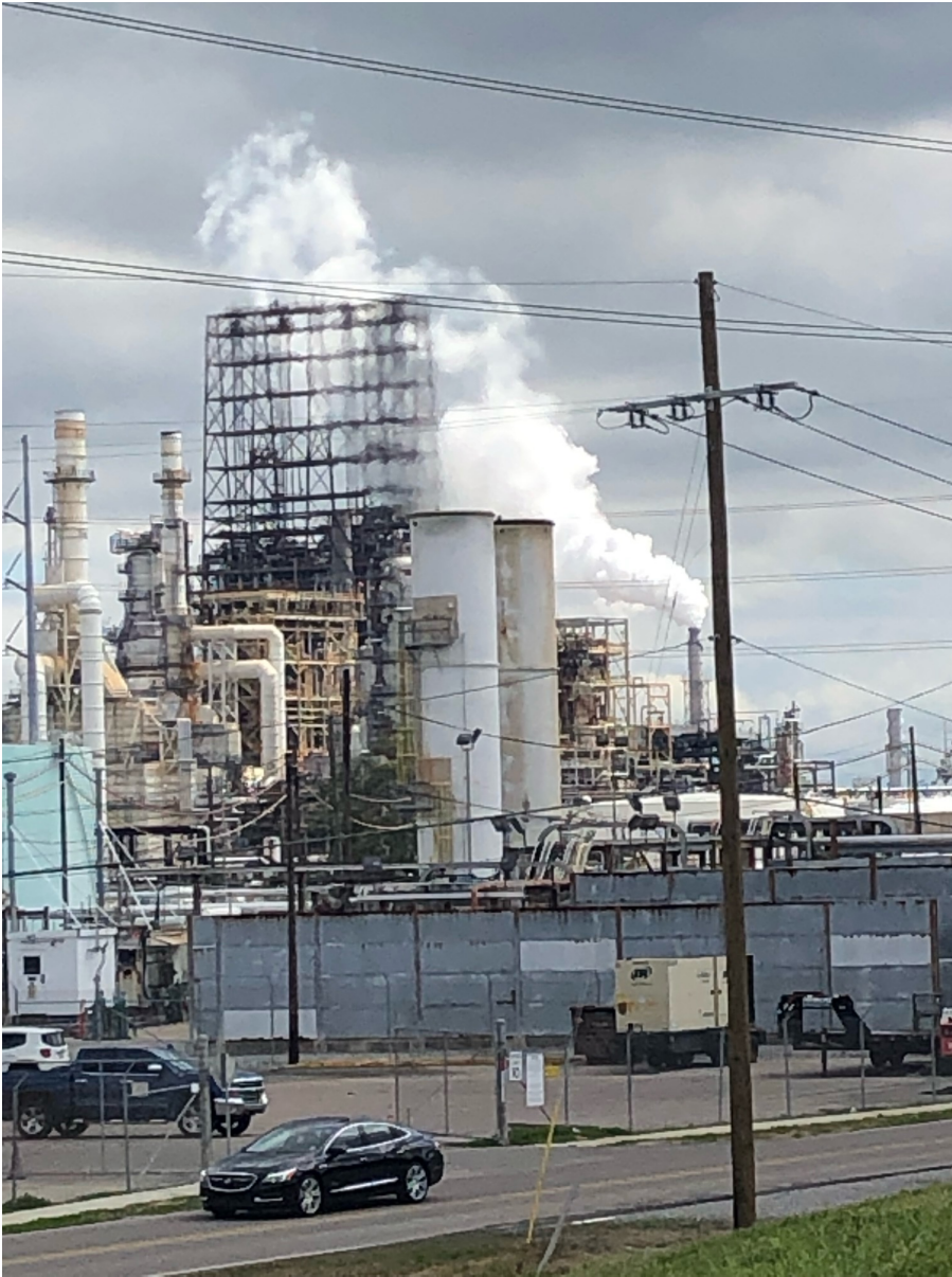
Figure 12: Pole Outside Facility, 2022
