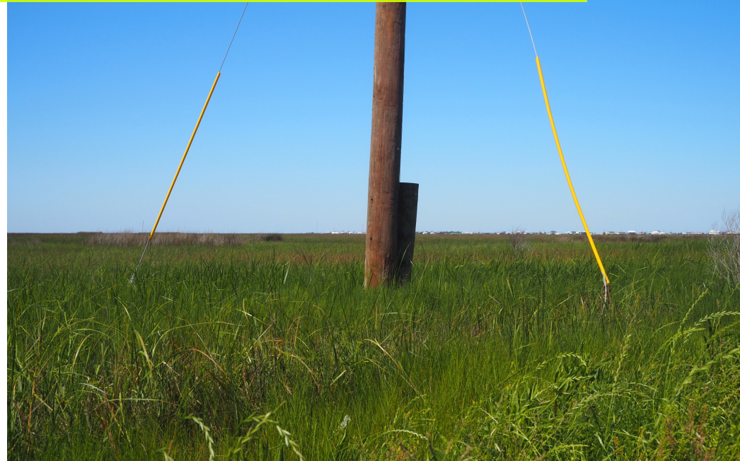
Figure 7: Pole with Guylines and Lashed Base, 2024
