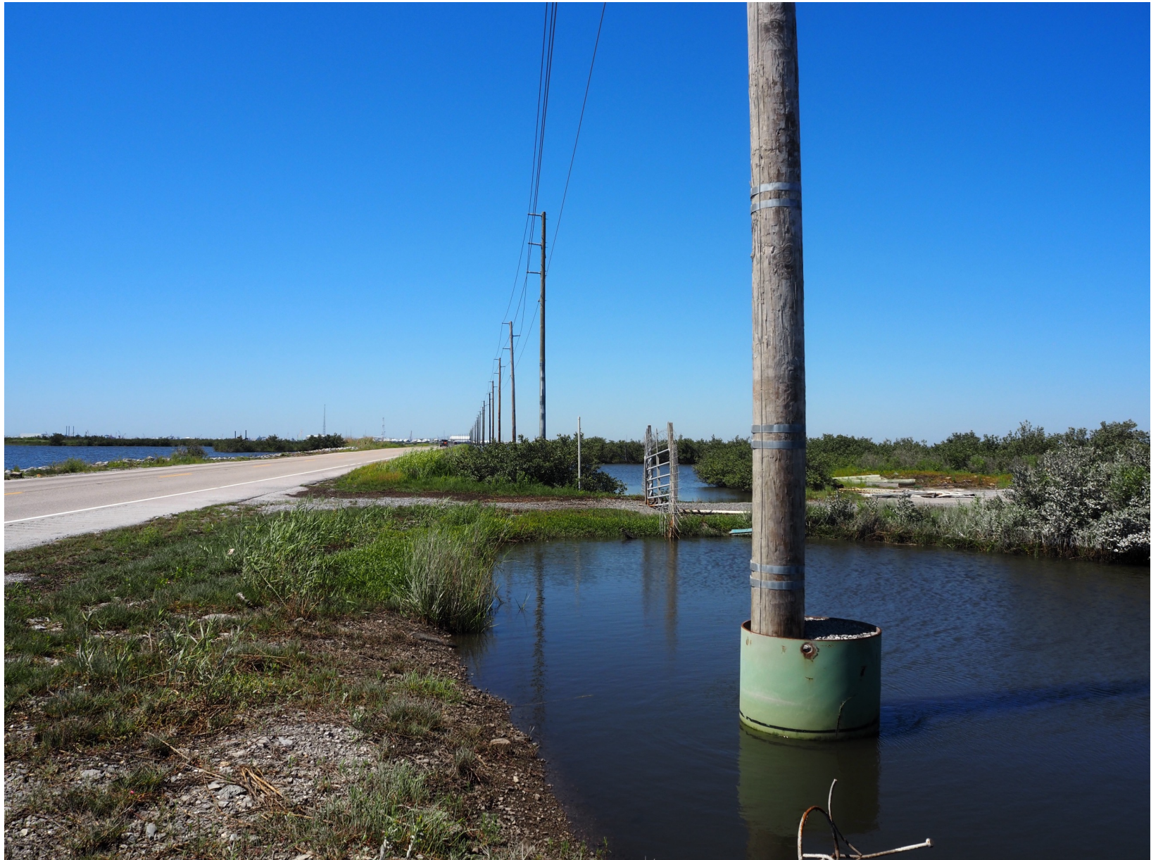
Figure 9: Pole with Steel Caisson, 2024
